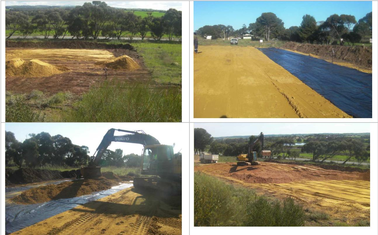
**Figure 3: Tailing Storage Facility - Trial Covers Construction Sequence**
