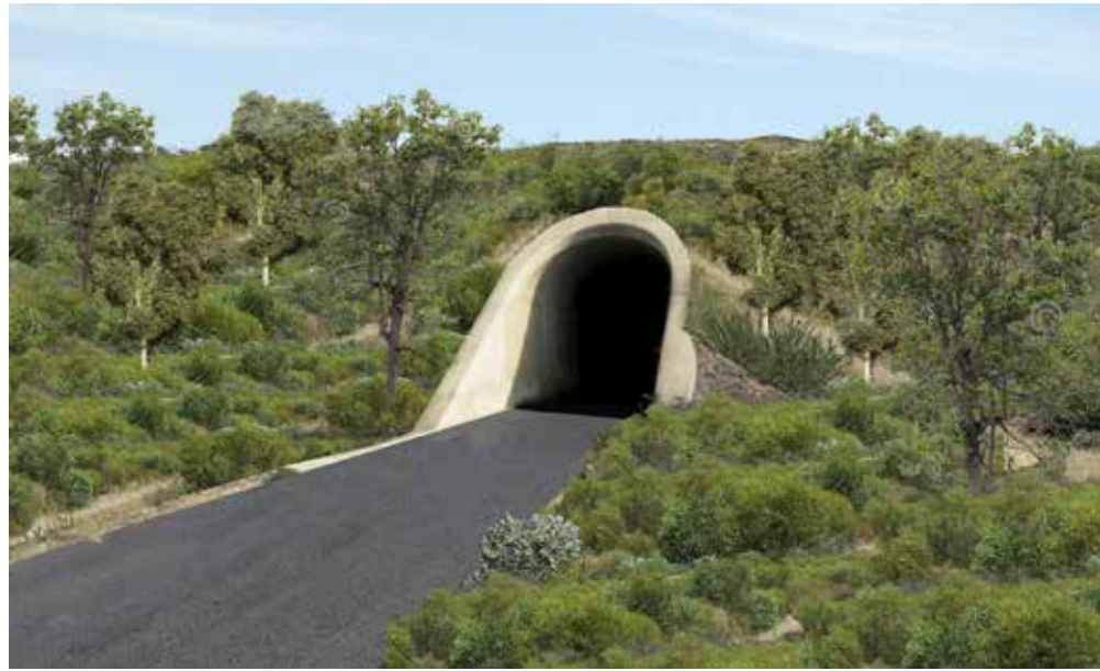
Mine Entry Portal
