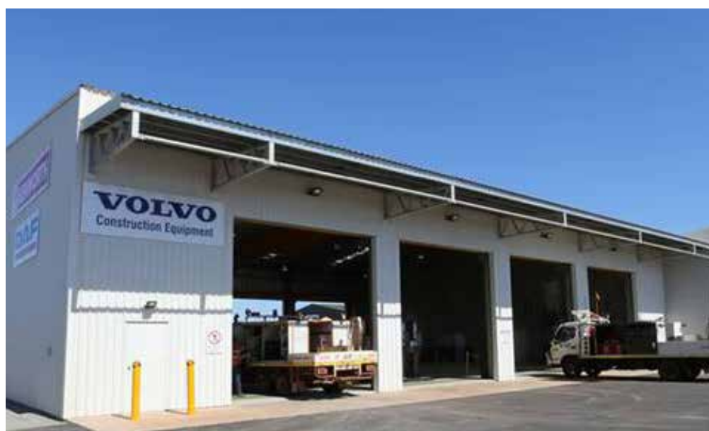
Vehicle Maintenance Workshop
