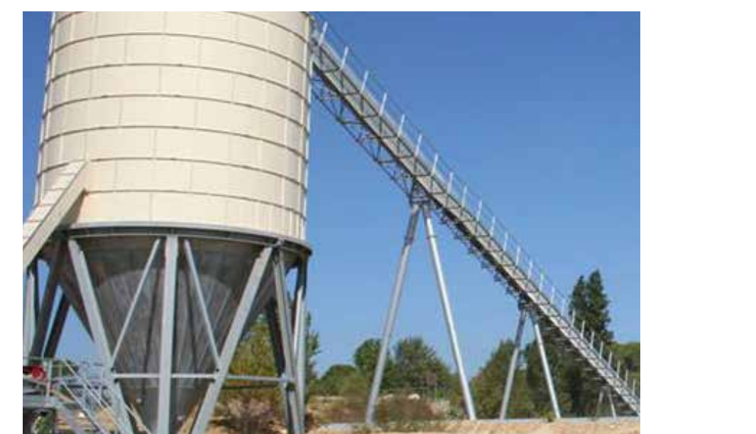
Ore Silo and Conveyor from Run of Mine
