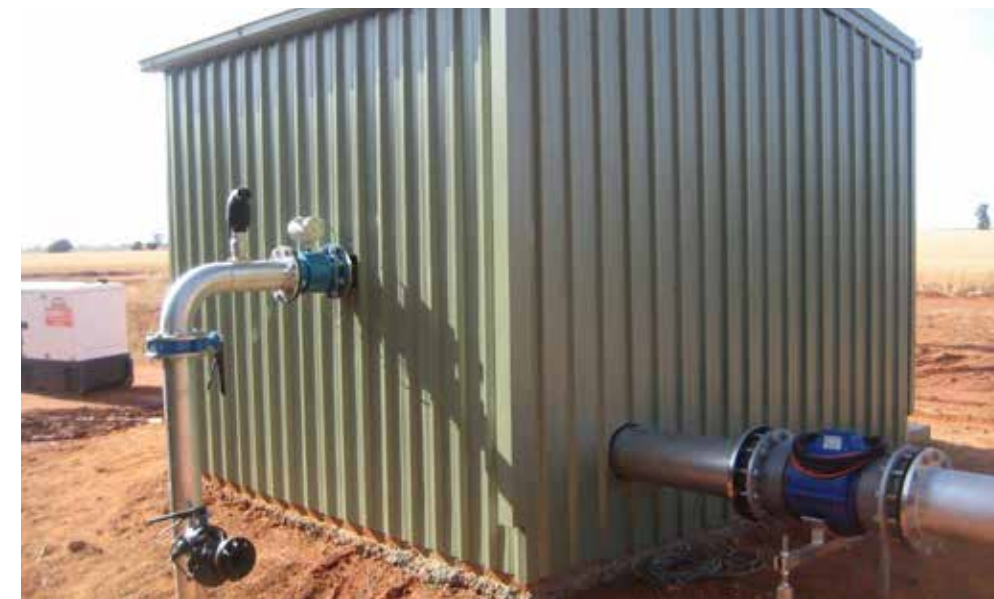
Dam Pump Shed
