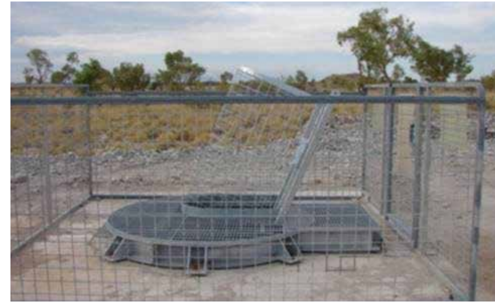
Emergency Exit Shaft
