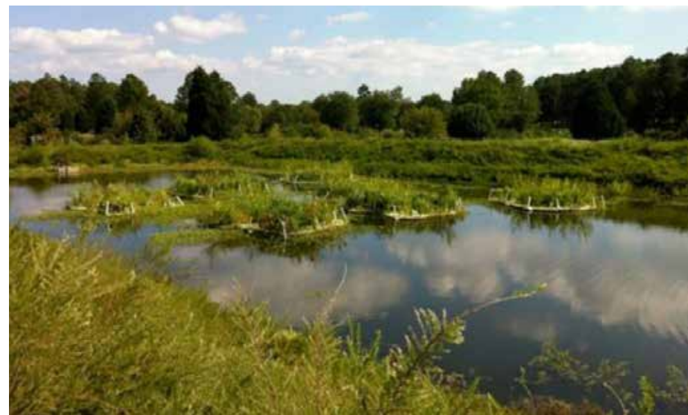
Mine Water Storage Dam
