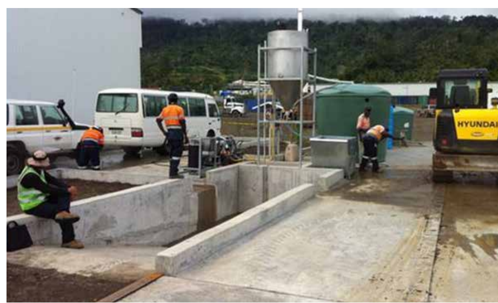
Vehicle Wash Pad
