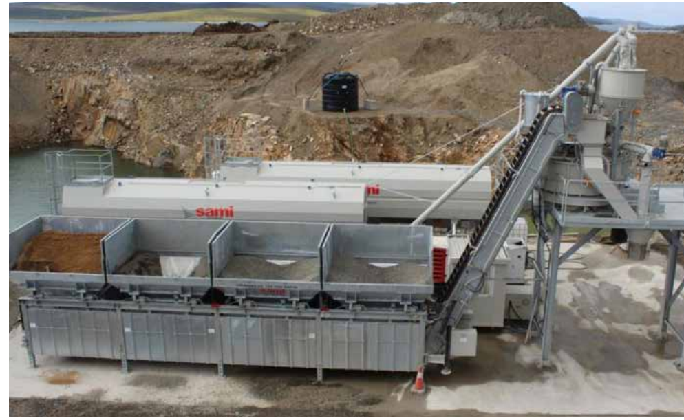
Concrete Batching Plant
