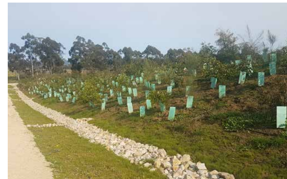
On-site Rock Lined Swale
