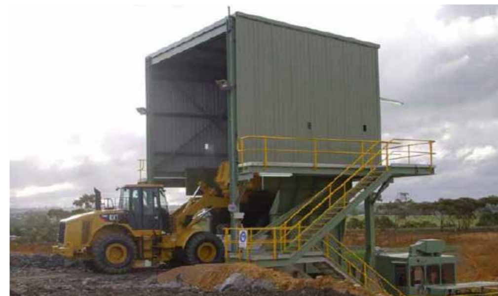
Enclosed loading bay
