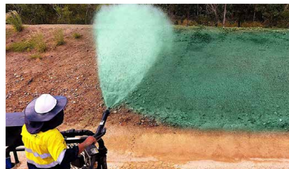
Hydromulching of landforms
