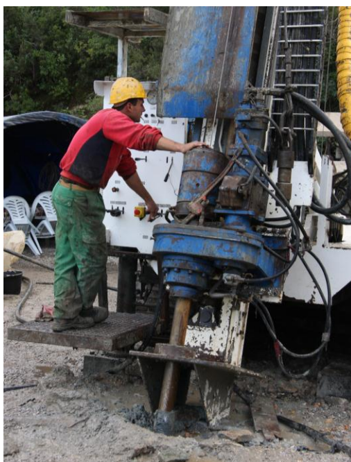
Drilling at Tala Hamza
