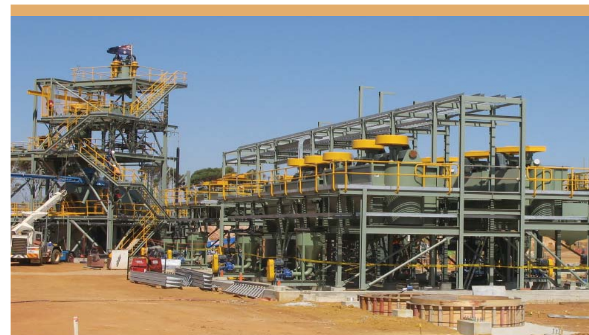
Process plant construction - grinding and flotation sections.
