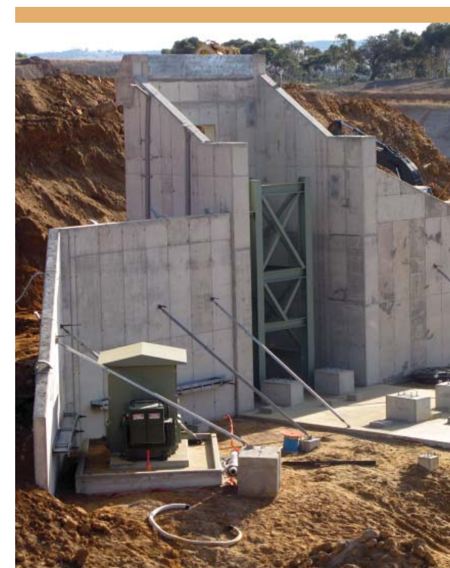
Angas crusher station construction.
