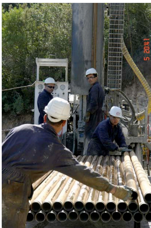
Spektra drill crew at work TH006
