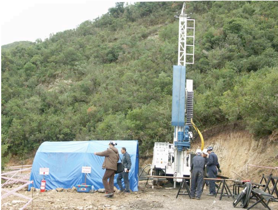
Spektra drill rig on location Tala Hamza (drilling TH006)
